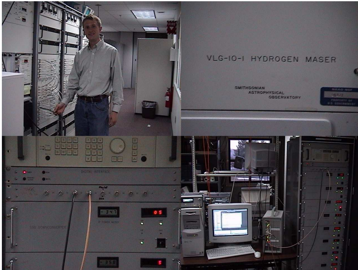
Figure 4.16: The GBT receiver system. Upper Left: Andrew Poulsen holding the 3.6 meter signal cable as it enters the GBT receiver converter racks. Upper Right: All local oscillators are synchronized with a reference signal generated by this hydrogen maser rack. Lower Left: Output of the spectral processor. The GBT signal is carried by the right cable and the reference signal by the left. Lower Right: After leaving the Spectral Processor, the signals directly enter the DSP.
